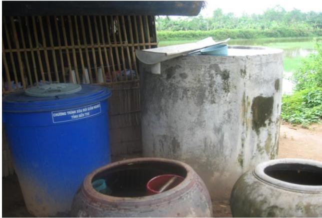
This rural house in Ben Tre Province uses a concrete tank to collect fresh rainwater. The tank doubles as a cyclone shelter during the wet season because it is the only structure solid enough to provide sufficient protection against hard objects carried by the wind: *pers. comm.* October 2010, Nguyen Van Kien
