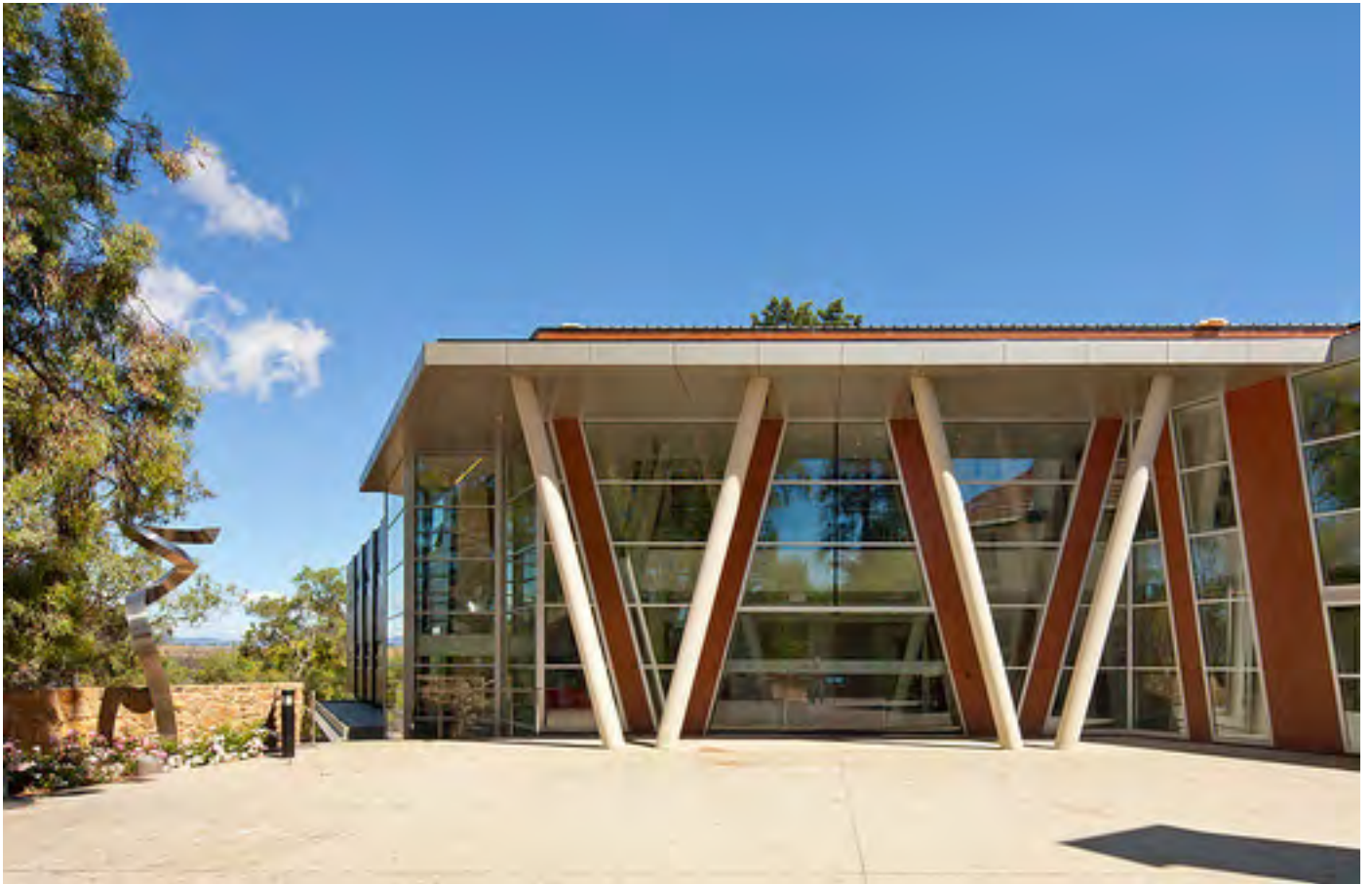
JG Crawford Building
