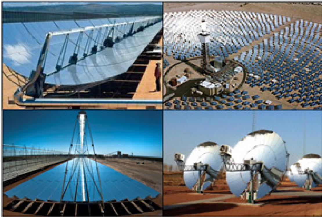
Figure 3. Different designs of Concentrated Solar Power plants. Top left: parabolic trough (Solar Millennium, 2018); top right: central tower receiver (Sandia National Laboratories, 2018); bottom left: linear Fresnel (Laird, 2012); bottom right: Parabolic dish with Sterling engine (Coventry and Andraka, 2017).
